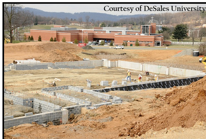
Figure 1: Footing Excavation and Constructed Foundation Walls
